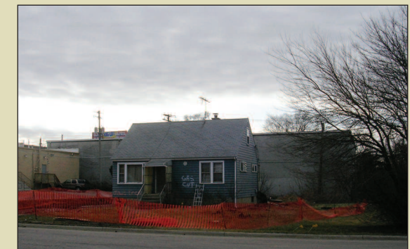
Another old building bites the dust on National property at 1112 S. Stewart, across the street from the newly renovated McDonald's at Stewart and Roosevelt Road.
